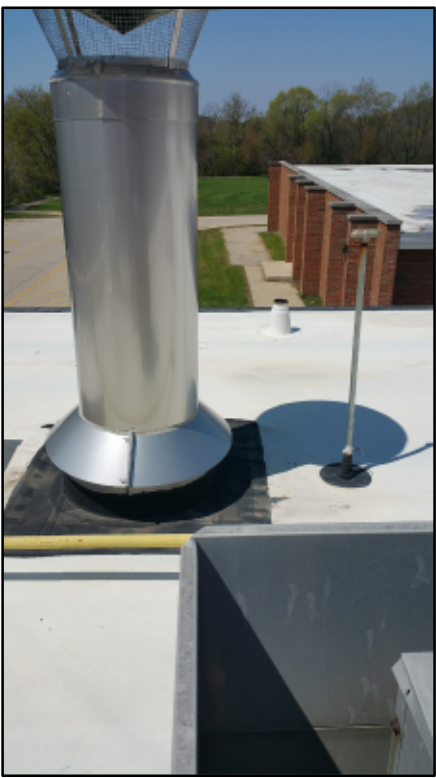
20 STACKS AT BOILER ROOM
