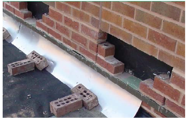
Photo 3 Flashing Installed in Alternating Sections
