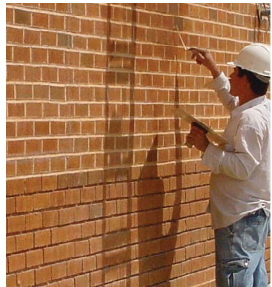
Photo 2 Repointing Mortar Joints
