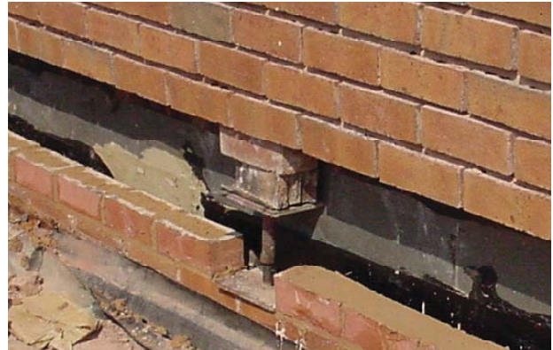
Photo 4 Flashing Installation Using Temporary Support
