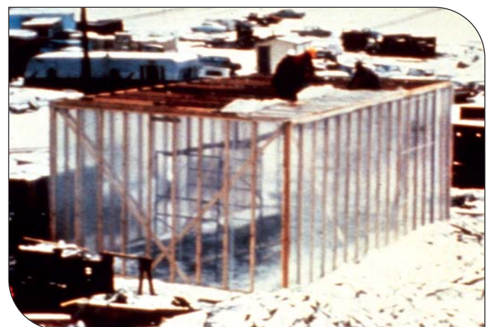
Figure 4. A temporary shelter protects the mortar preparation area from rain and snow. (IMG24817)
