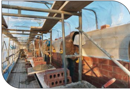
Figure 5. Enclosure and heating of a work area protects materials, workers, and installed masonry from severe weather. (IMG12508)
