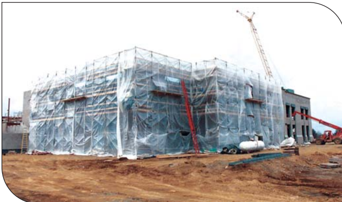
Figure 1. Masonry construction can proceed through winter months if an effective cold weather construction program is adopted. (IMG12504)
