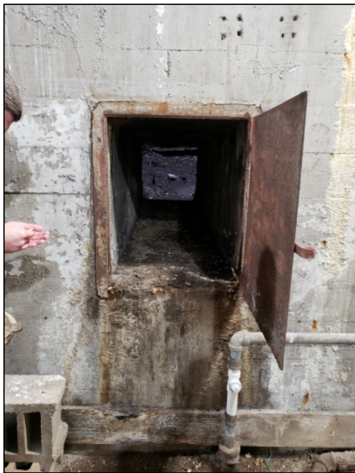
4 ASH DOOR TO REPLACE SCALE: NONE
